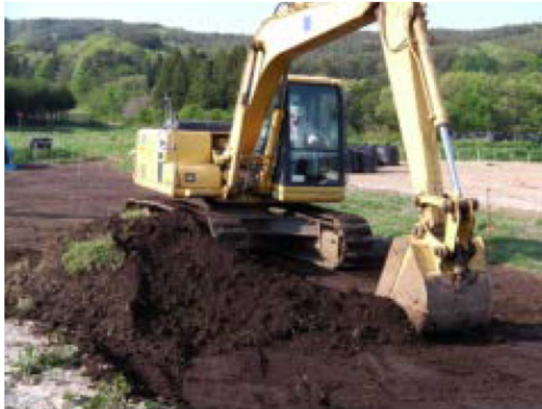
Stripping topsoil method
