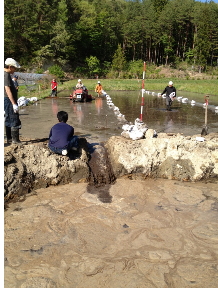
Flush out muddy water by tractor
