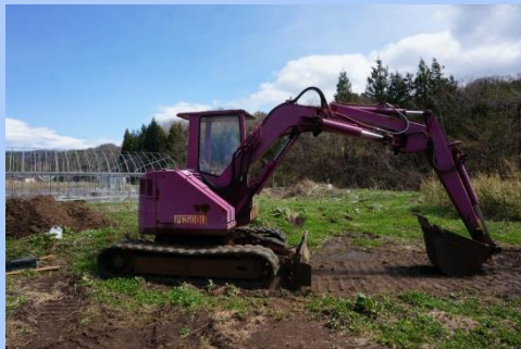
stripping the 5 cm top soil
