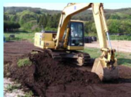
Stripping topsoil method
