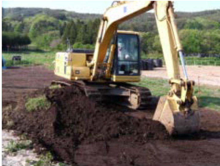
Stripping topsoil method
