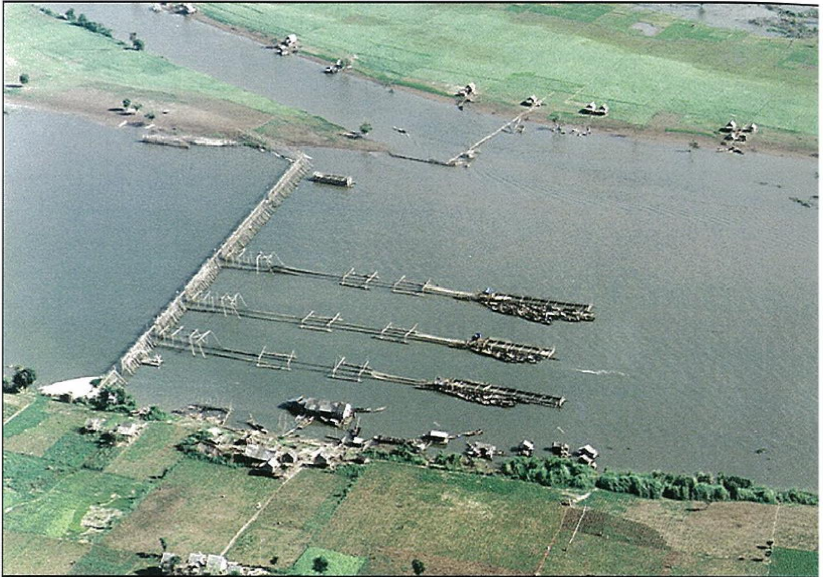
Fishing Int No. 9 in Kamnong Chhnang Barrage with 3 weir sorting plat
