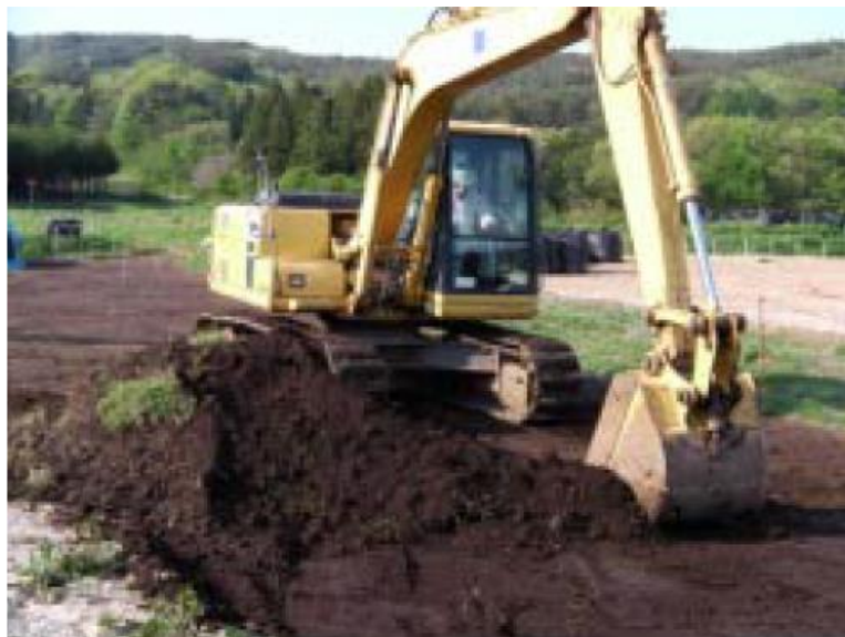
Stripping topsoil method
