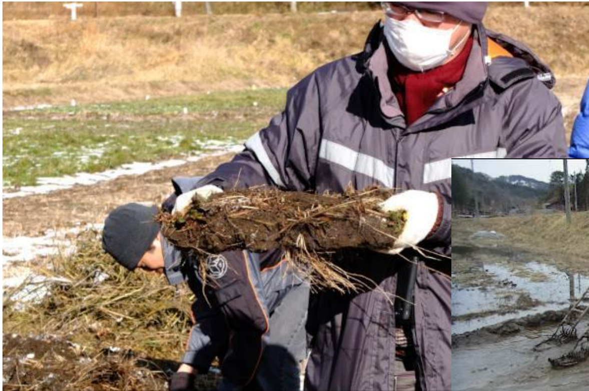
decontamination method by stripping frozen soil (2012.1.8)
