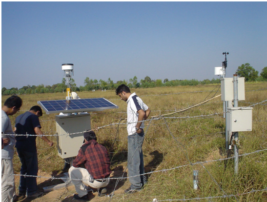
Fig. 1. Field Server installed on 2007 December 24
