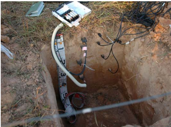
Fig.3 Installation of soil sensors
