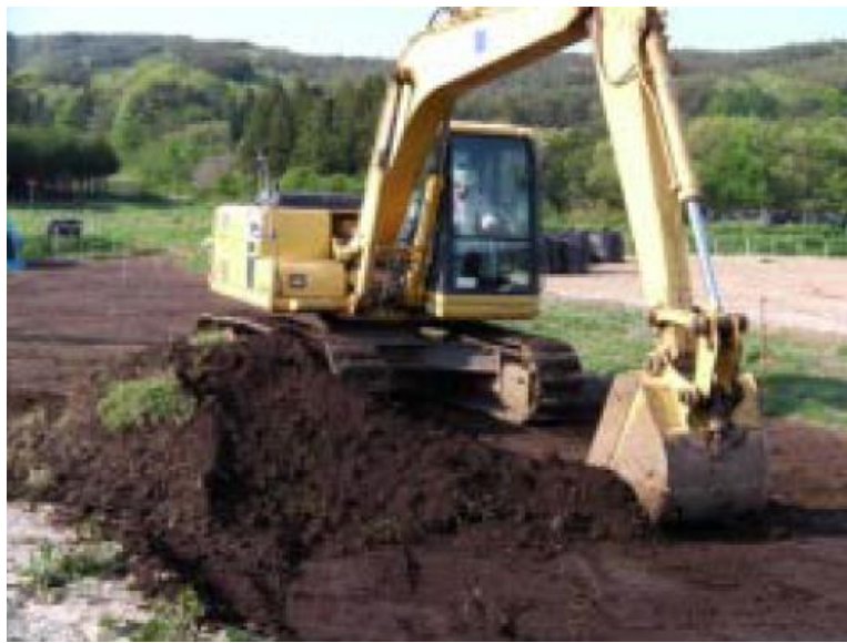
Stripping topsoil method
