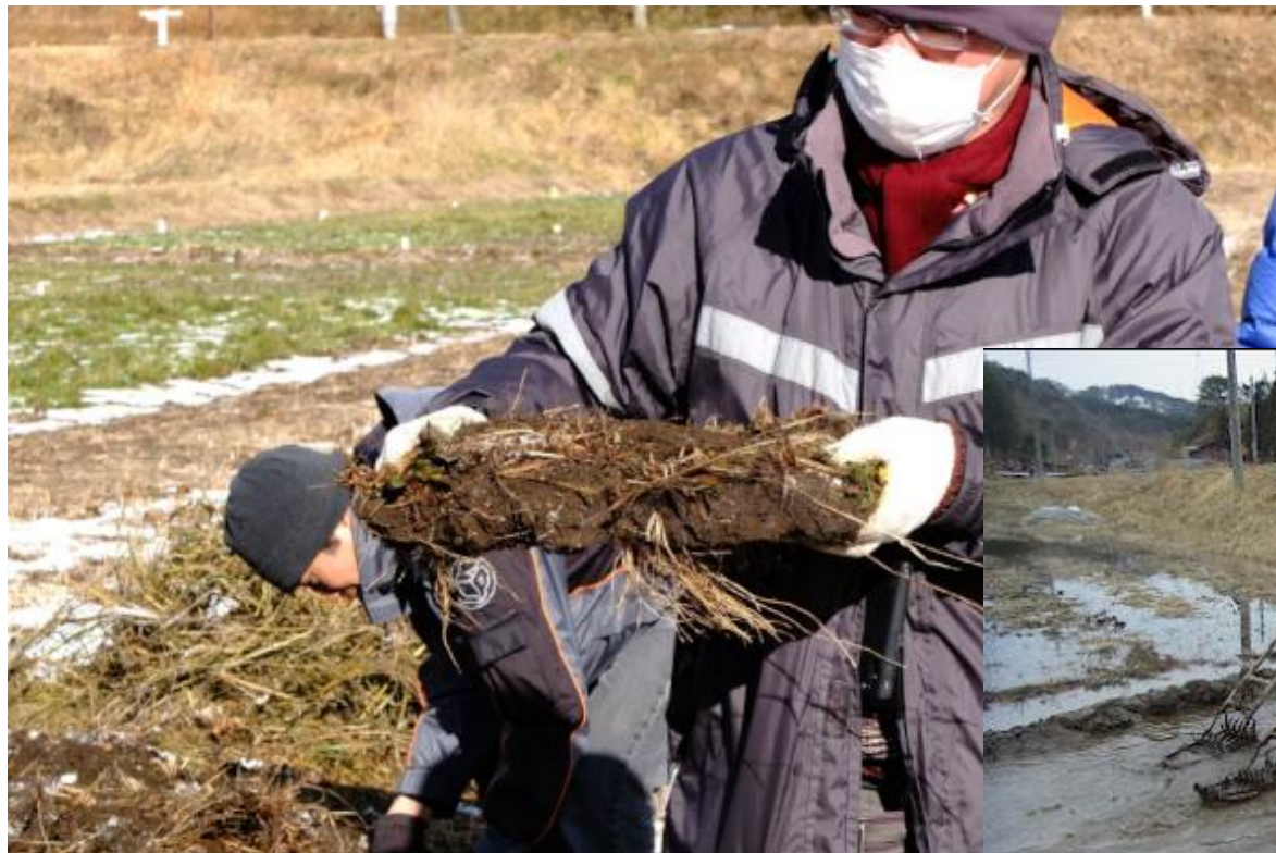
decontamination method by stripping frozen soil (2012.1.8)
