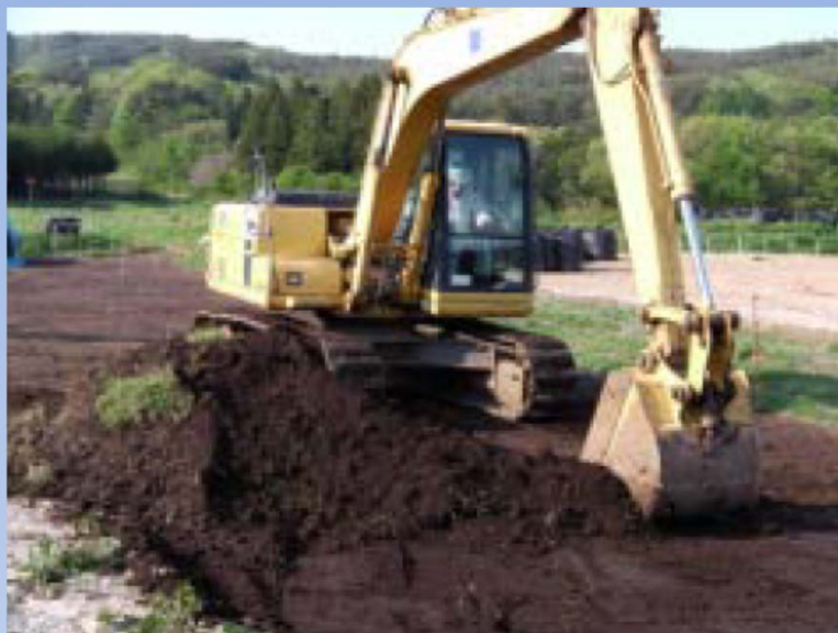
Stripping topsoil method
