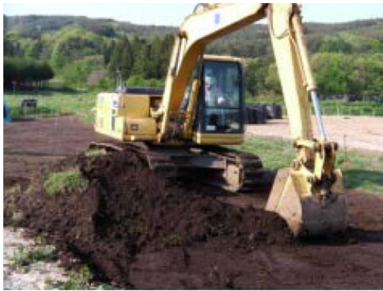
Stripping topsoil method
