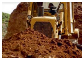
Farmland is being decontaminated by removing the topsoil with heavy machinery.
